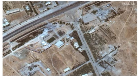
A satellite image shows significant damage to buildings at Iran's Kermanshah Missile Facility after repeated Israeli Strikes on the site. Maxar Technologies
